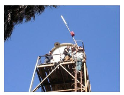
Figure 11.24: Implementation of node over a water tower in Batuco, Metropolitan Region, providing backhaul to Cabrati telecenter.
