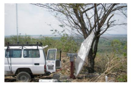
Figure 11.34: El Baúl antenna installation. Actual elevation was 1° upward, since the antenna has an offset of 22.5°.
