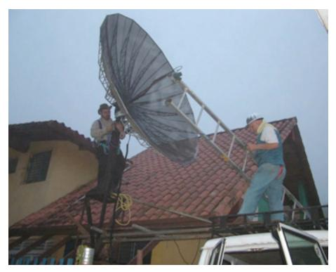
Figure 11.30 shows the disassembly of the mesh reflector.
