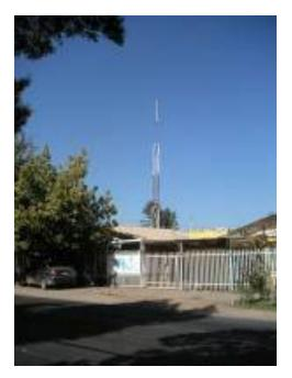
Figure 11.21: Node in southern Santiago, consisting of a 15 m tower, a Trevor Marshall 16+16 antenna, and 30 clients. The node is connected to a downtown node more than 12 km away.
