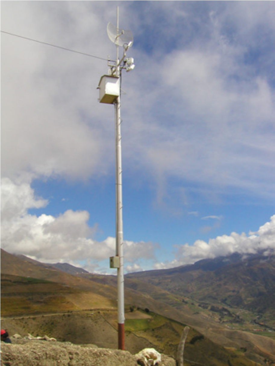
Figure 8.3: A simple self-supporting tower.
