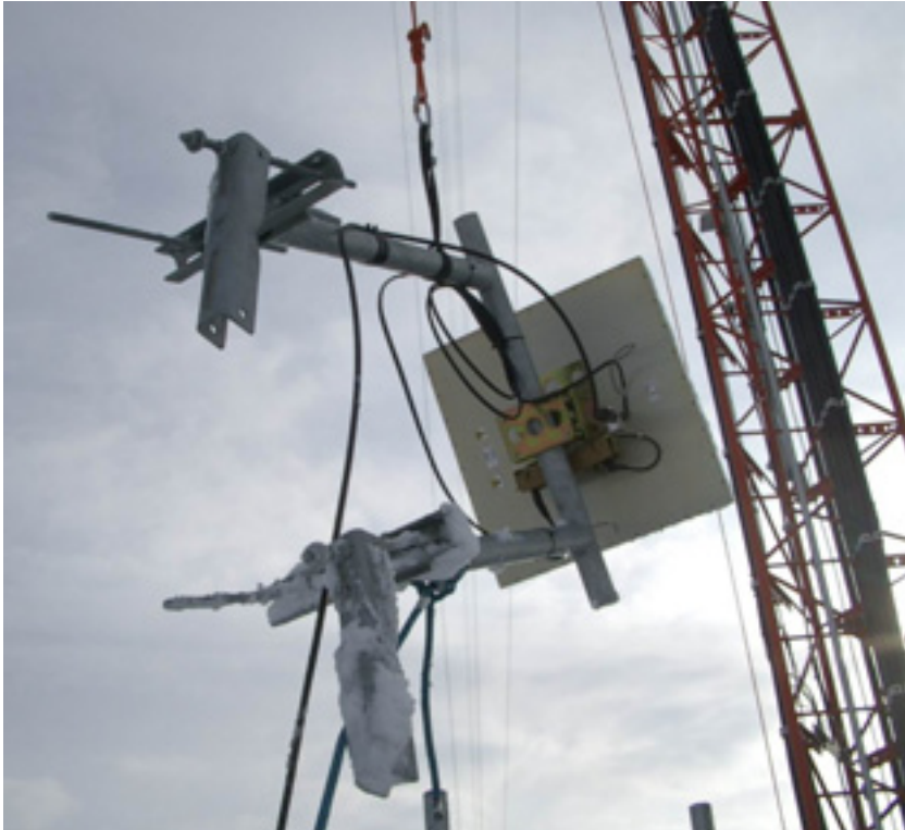
Figure 8.1: An antenna with a standoff bracket being lifted onto a tower.
