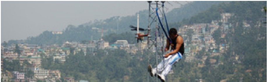
Figure 11.5: Dharamsala installer working on a tower
