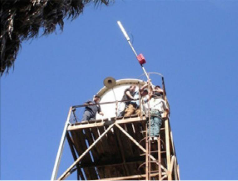
*Figure 11.24: Implementation of node over a water tower in Batuco, Metropolitan Region, providing backhaul to Cabрати telecenter.*
